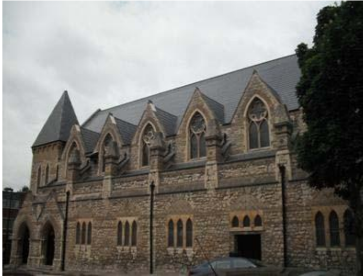
St Silas Church, Pentonville showing integrated solar PV tiles
