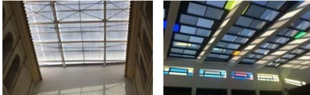
Examples of glass substitution by PV glass with shading properties (c-Si)
